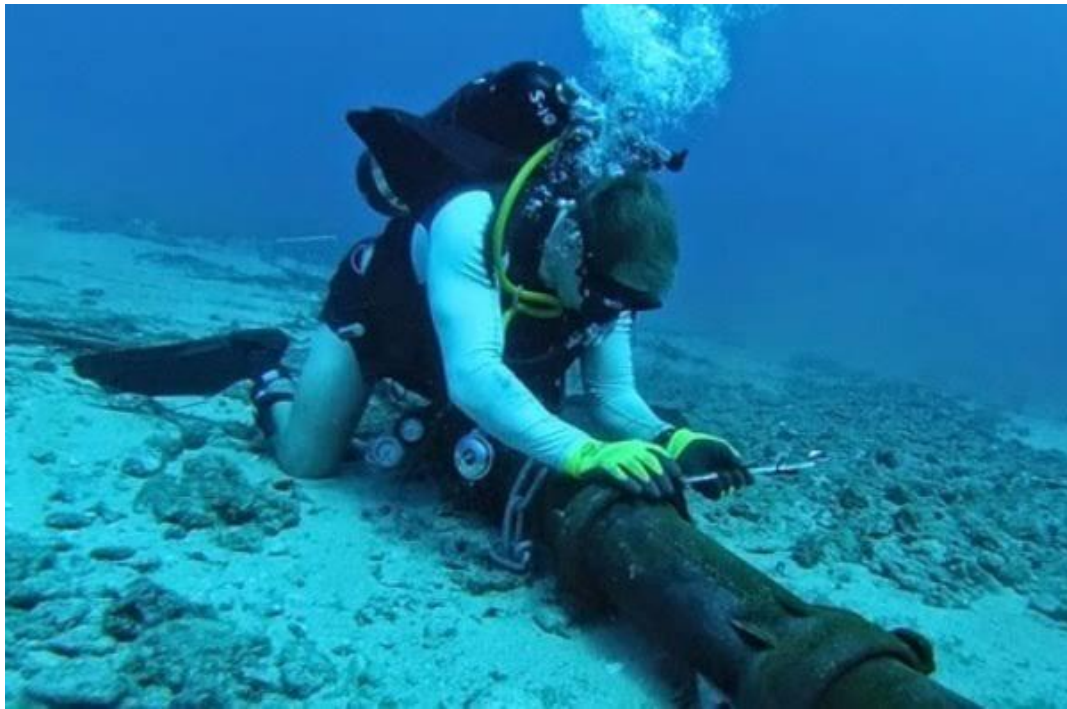
Figure 1. Subsea Pipeline Inspection
