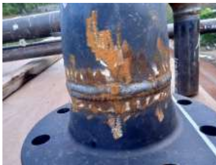
Figure 5 Surface results of side 1 CS welding
