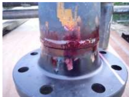
Figure 6 Application of penetrant liquid on side 1 CS
