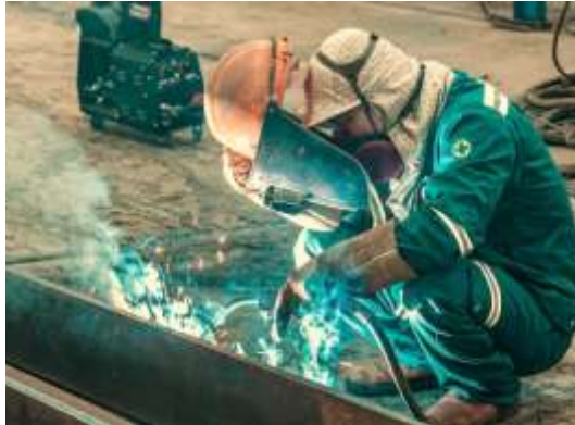
Figure 3. Welding Training Preparation
